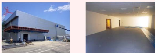
External and internal appearances of the Temporary Administration Office Building
