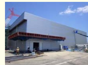
<External appearance of the Temporary Administration Office Building>
