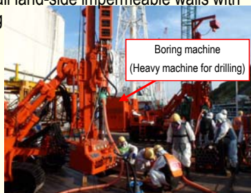
<Installation of frozen pipes of land-side impermeable walls with frozen soil>
