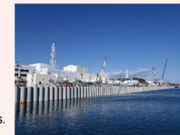
Installation status of impermeable walls on the sea side
