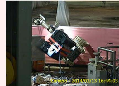
Status of remote-control robot falling down
