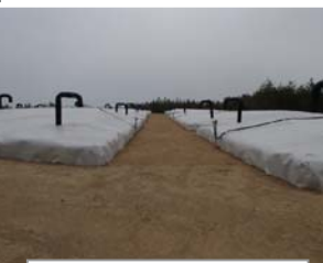
Temporary trimmed trees storage pool
