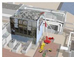
Removal of rubble on the roof of the Reactor Building
