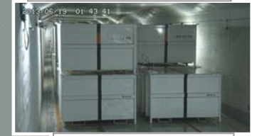
Solid waste storage
