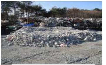
Rubble (outdoor accumulation)
