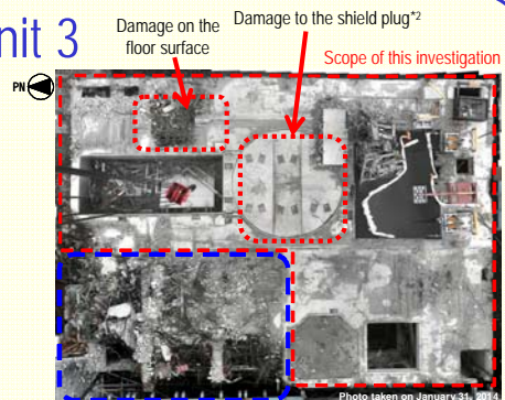
Confirmed by the status investigation immediately after the earthquake * Full view produced by integrated photos of investigation <Investigative result of operation floor>
