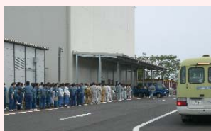
External view of the entrance control facility
