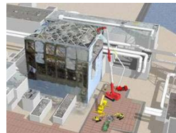
Removal of rubble on the roof of the Reactor Building
