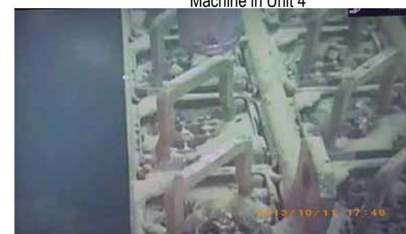
Before absorbing rubble
