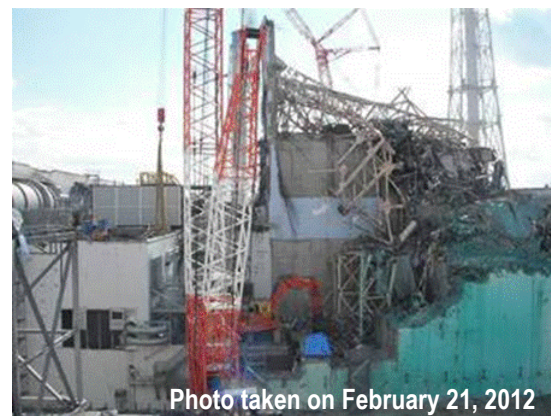
Before removing large rubble
