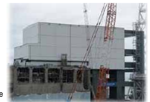
Figure 6: Unit 4 with a cover for fuel removal installed
