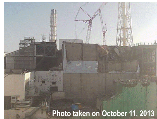
After removing large rubble
