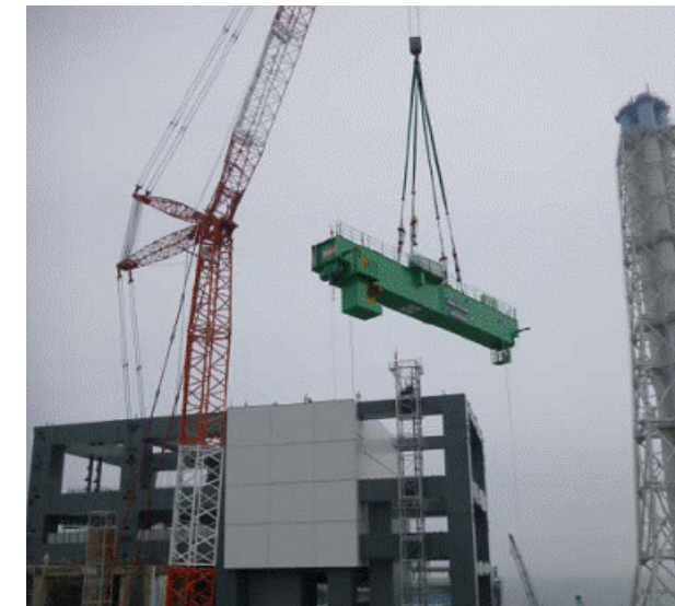
Figure 5: Lifting of overhead crane for Unit 4
