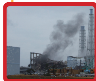
11:01 Hydrogen explosion in the Unit 3 reactor building
