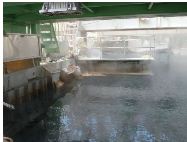
Conditions at the Unit 4 spent fuel pool, photographed June 29, 2011
