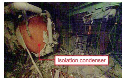
Damage to an isolation condenser
