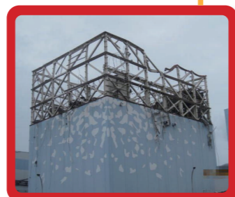
15:36 Hydrogen explosion in the Unit 1 reactor building (panel opened on the side of the upper part of Unit 2 reactor building)
