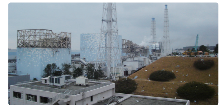
Fukushima Daiichi Nuclear Power Station, after the accident (from left to right, Units 1, 2, 3, and 4; photographed March 16, 2011)
