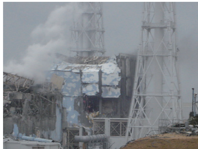
Unit 4 reactor building after the hydrogen explosion
