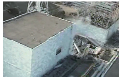
Panel on the side of the upper part of the reactor building opened with the hydrogen explosion at Unit 1
