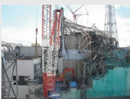
Before the removal of large debris
