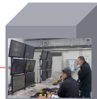
Remote operations room (Main Office Bldg.)
