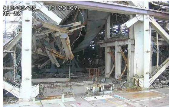
After removal of X-brace
