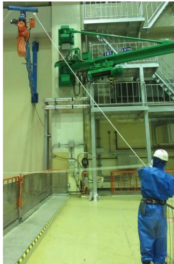
Installing temporary diesel generator and jib crane at Fukushima Daiichi
