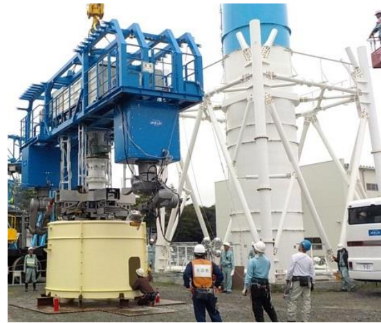
Remotely operated dismantling equipment (Left), Mock-up exhaust stack (right)
