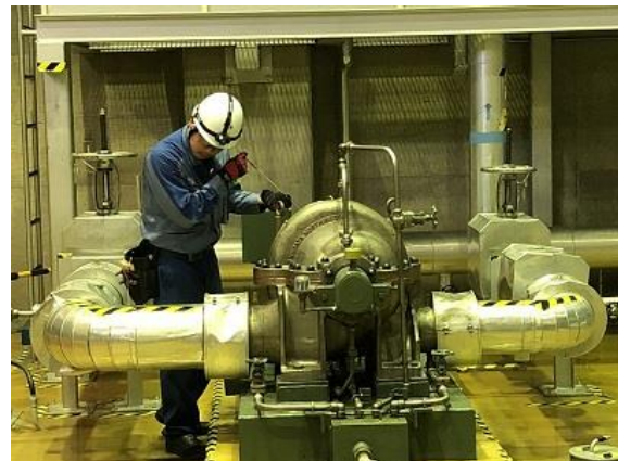
Field skill competition (pump startup check)
