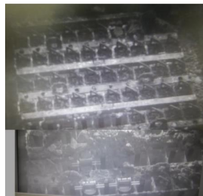
New fuel after rubble removal (June 8)
