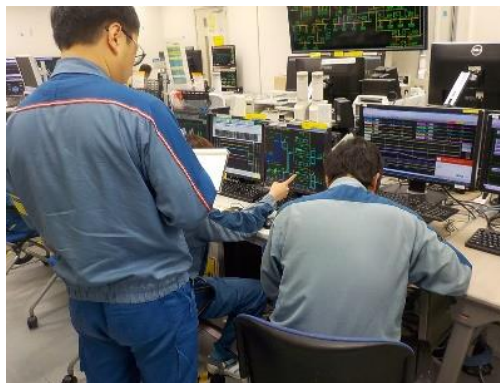
Main Control Room
