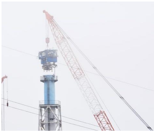
Checking equipment fit on top of exhaust stack
