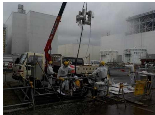
After kaizen: Lifting pump with Unic crane truck
