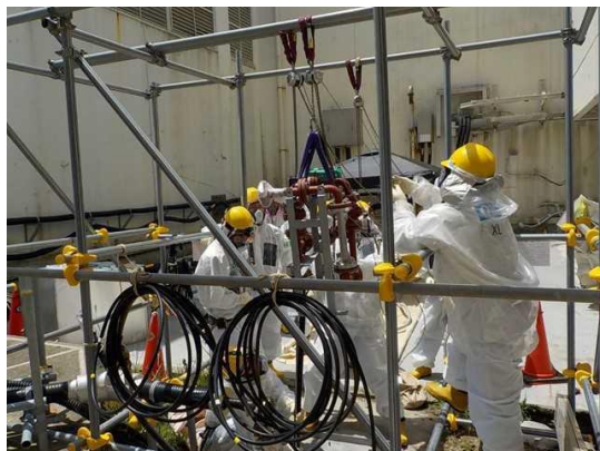
Before kaizen: Lifting pump using hoisting frame
