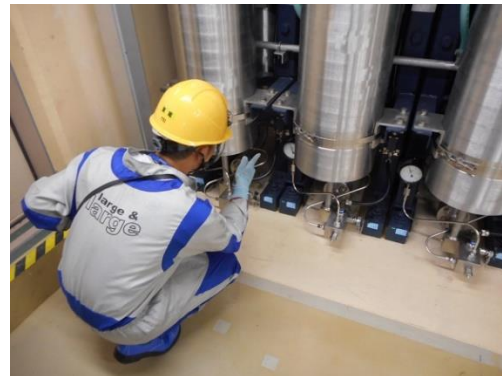
Reactor scram check test during HEMP (Field deployment)
