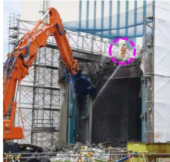
Before kaizen: Workers spraying water
