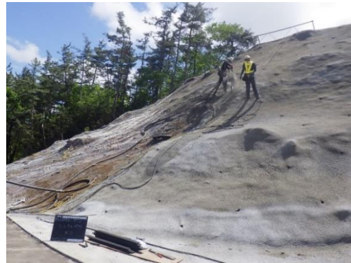
Mortar spraying
