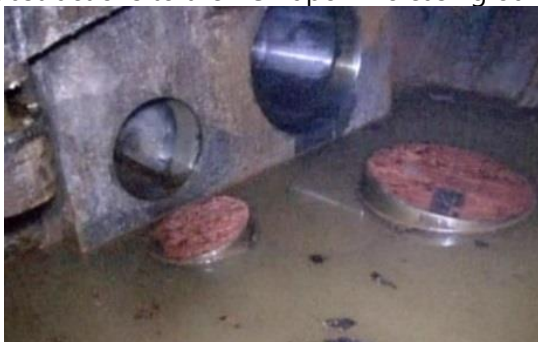
Holes cut in outside door
