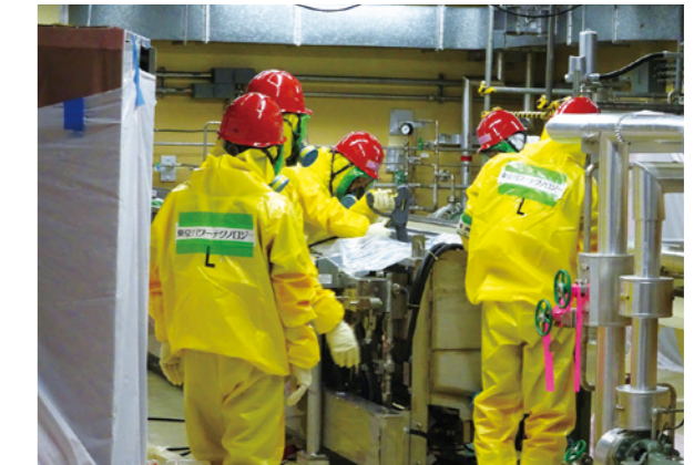
Decontamination during the Decommissioning of the Fukushima Daini Nuclear Power Station
