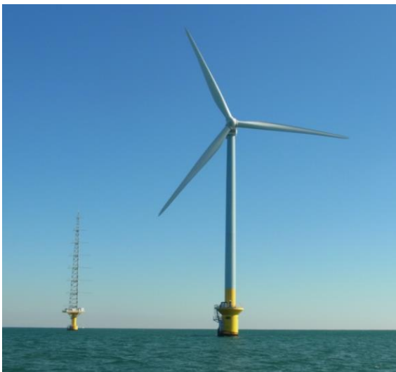
Offshore wind power generation test facility and wind-measuring tower
