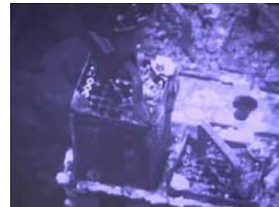
Fuel removal work
