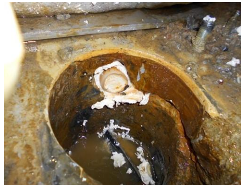
Floor funnel sealed using filler material
