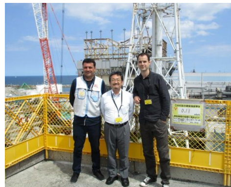
Unit 1 reactor building
