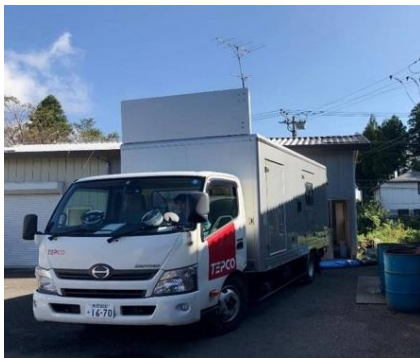
Supplying power using power supply trucks from Kashiwazaki-Kariwa
