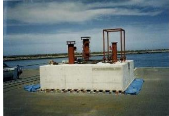
Wave meter installed in 2001
