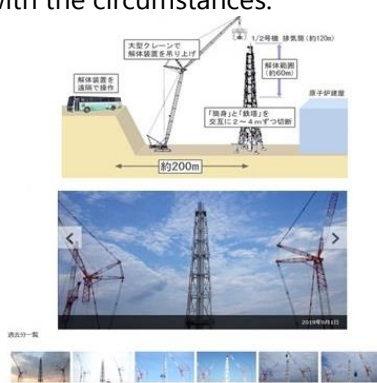
Unit 1/2 exhaust stack dismantling page
