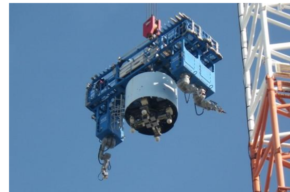
Lowering a piece of the exhaust stack
