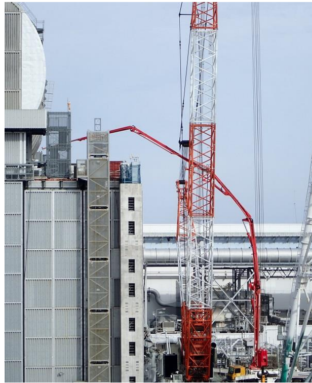
Concrete pump truck
