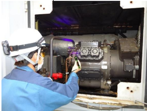
Detecting refrigerant leaks by injecting a florescent agent into air-conditioning freezers (Left: Checking for freezer coolant leaks, right: Goggles and UV light used to check for fluorescent agent leaks)
