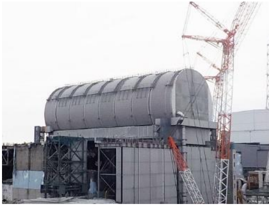
Completed domed roof for fuel removal
