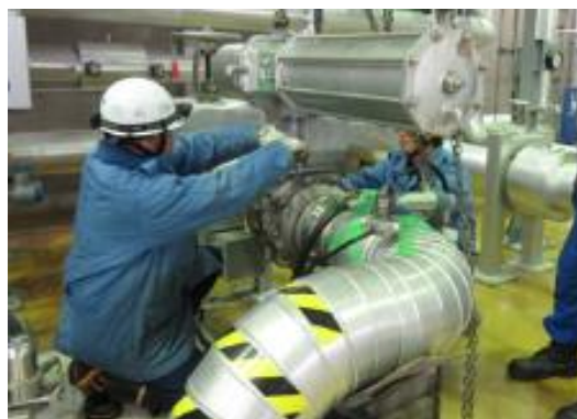
Right: Valve/drive mechanism inspections (hoisting drive mechanism)
