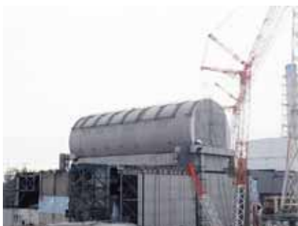
Completing domed roof of Unit 3 fuel removal cover (Feb. 23)
