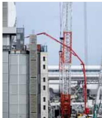
Training in using concrete pump trucks to inject coolant into Unit 3 (March 20)
