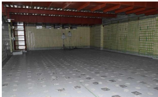
Prior to renovation (old process computer room) After renovations (Anchors being installed to erect shielding walls)
