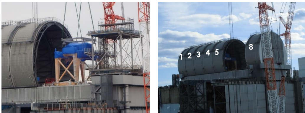
Domed roof installation (Left: Crane installation, Right: Domed roof segment installation)
