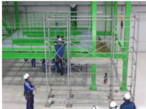
Training on assembling and disassembling scaffolding to experience the dangers associated with such tasks
