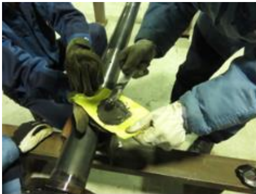
Pipe duct repair training
