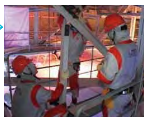
Addition of copper materials (Kashiwazaki-Kariwa Nuclear Power Station)
