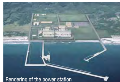
Rendering of the power station Higashidori Nuclear Power Station (Aomori Prefecture)
