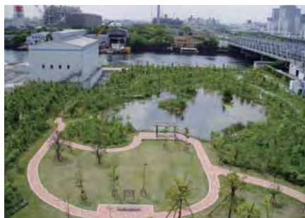
Biotope at the Shinagawa Thermal Power Station
