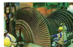
Turbine inspection and restoration (Unit 4)
