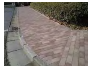
Pavement made of non-fired bricks
