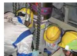
Seismic reinforcement of pipe supports (Unit 3)
