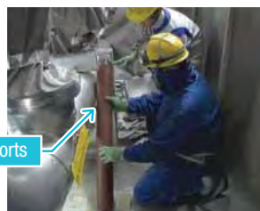
Reinforcement of pipe supports (Kashiwazaki-Kariwa Nuclear Power Station)
