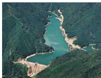
Imaichi Dam (construction site of the Togawa Hydropower Station)
