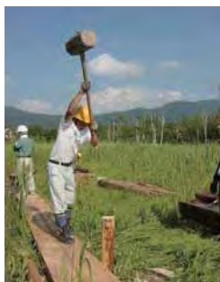
Maintenance of the wooden walkway
