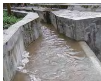
Power generation facility (sand basin)
