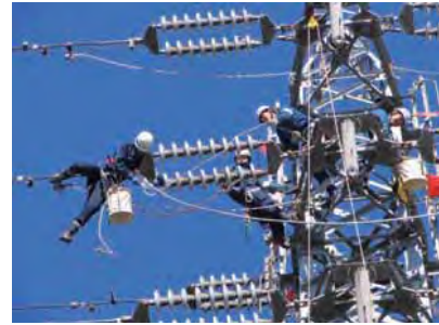
Accident recovery training atop a transmission line tower
