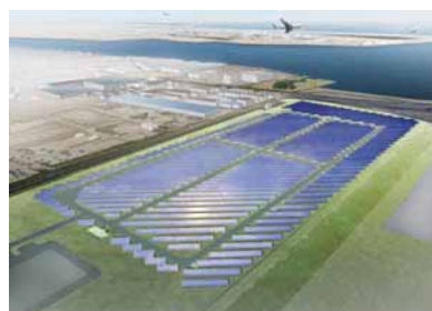
Rendering of the Ukishima Solar Power Plant
