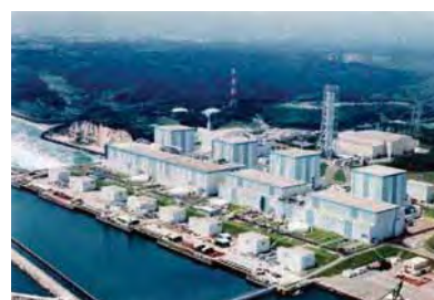
Fukushima Daini Nuclear Power Station (Fukushima Prefecture)
