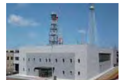
Seismic-isolated building at the Kashiwazaki-Kariwa Nuclear Power Station
