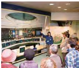
Service hall in a nuclear power station
