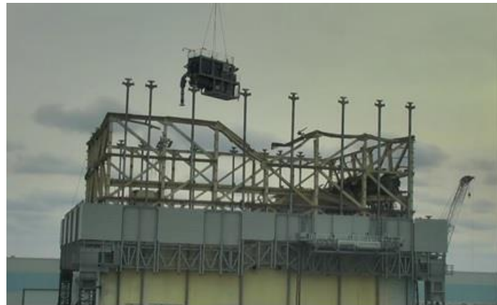
Insertion of rubble suction equipment into Unit 1
