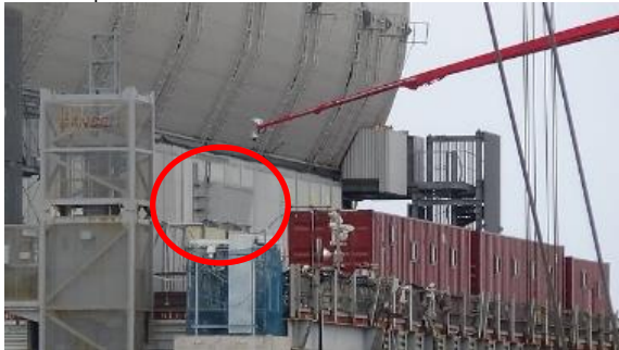
Unit 3 coolant injection receptacle
