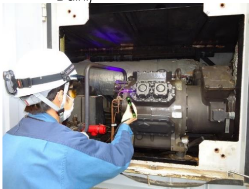
Detecting refrigerant leaks by injecting a florescent agent into air-conditioning freezers (Left: Checking for freezer coolant leaks, right: Goggles and UV light used to check for fluorescent agent leaks)
