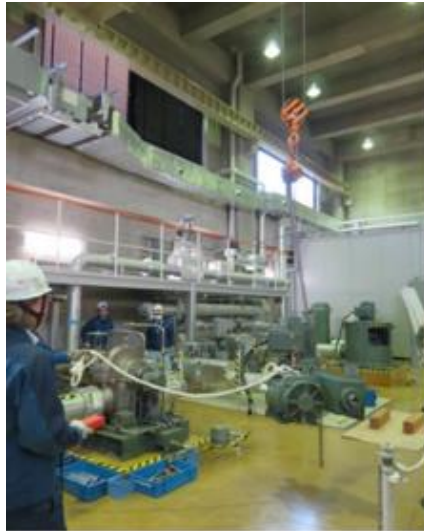
Pump disassembly inspection (motor hoisting)
