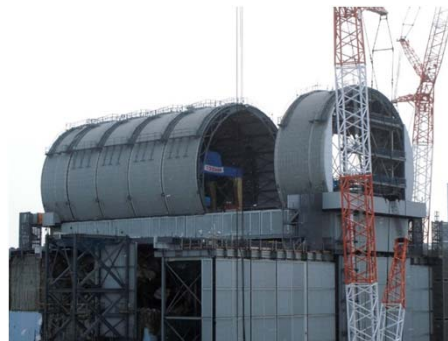
Unit 3 Fuel removal cover (domed roof) installation (December 12)
