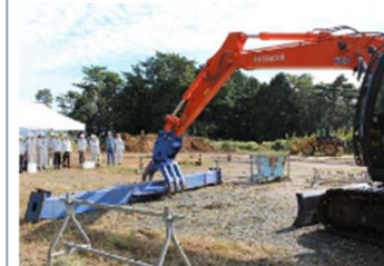
In-house debris removal training (Fukushima Daini)
