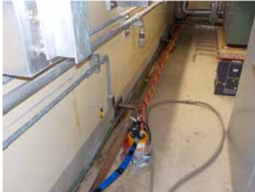
Installation of automatic groundwater drainage line
