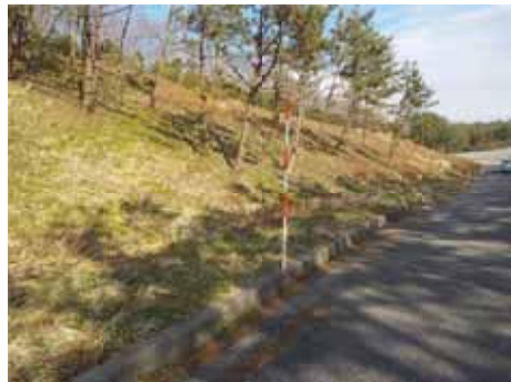
Before asphalt paving
