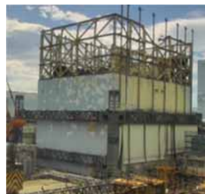
Conditions after removal of pillars and beams
