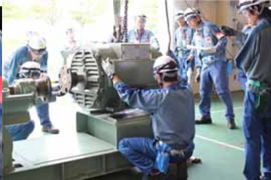
Motor replacement training
