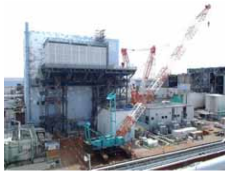
Platform and anteroom construction (Photographed on May 9)
