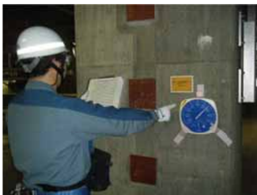
Installation of temperature and humidity gauges in cable tray areas
