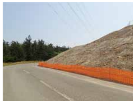
During construction of fire belt (after felling of trees)
