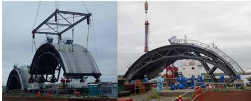
Unloading of the domed roof of the fuel removal cover
