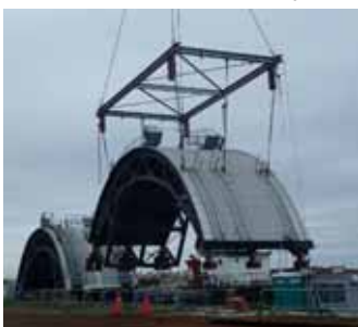
Arrival of Unit 3 fuel removal cover (June 27)
