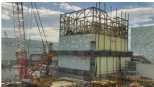
Completion of removal of the pillars and beams from the Unit 1 building cover (May 11)
