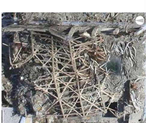
Refueling floor right after accident (photo taken in March 2011)
