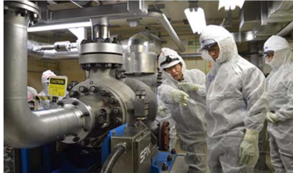
Field tour for the mayor of Kashiwazaki City (Unit 7 high-pressure alternate coolant injection system pump installation)
