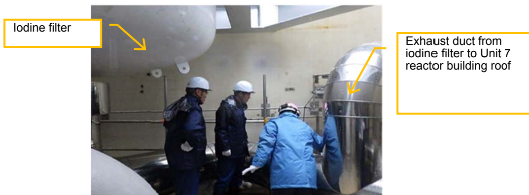
Field tour for the mayor of Kashiwazaki City (Equipment installation under iodine filter behind the Unit 7 filter vent shield)
