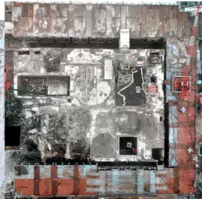
Refueling floor at the beginning of decontamination (photo taken in March 2014)
