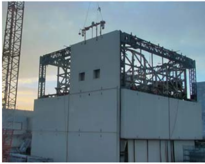
Removing wall panels
