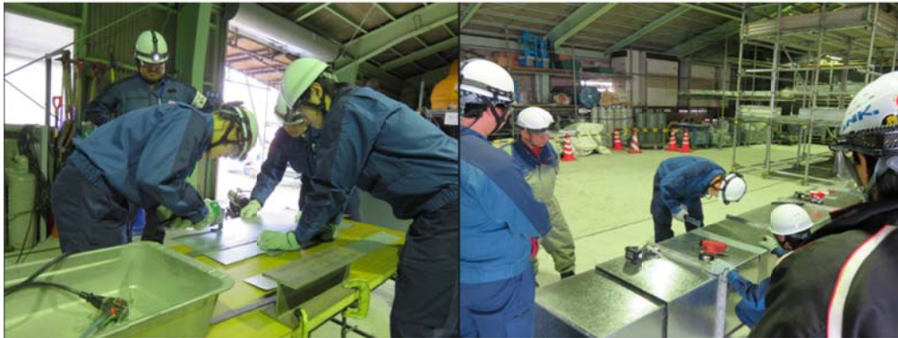
Training on repairing main control room air conditioning ducts (left: cutting out repair panels, right: installing rivets)
