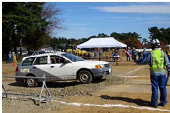
Kashiwazaki-Kariwa NPS team (left: slope building, right: confirming the vehicles can pass over the slope after the road repair)
