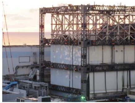
After removal of all wall panels
