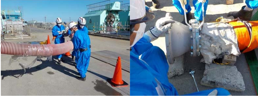
Training on laying temporary hoses (left: hose laying, right: connecting flanges)
