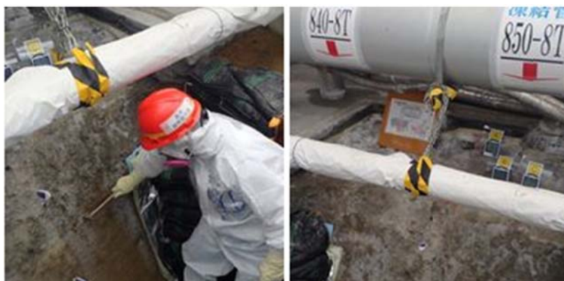
Visual check of the status of freezing of the land-side impermeable wall (from Facebook)
