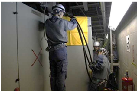
Connecting cables to power panels
