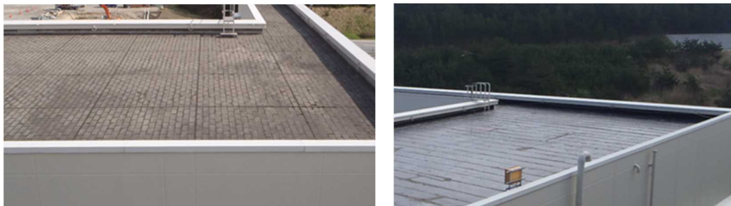
Removal of roof blocks from a building roof (left: before removal of roof blocks; right: after removal)
