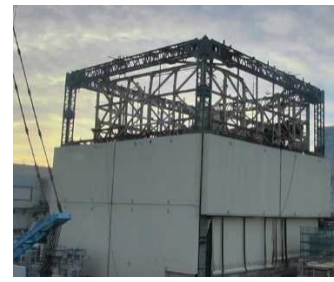
Removal of upper wall panels completed
