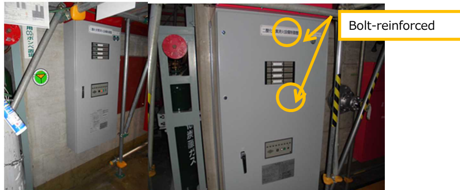
Emergency diesel generator prior to seismic reinforcement Emergency diesel generator after seismic reinforcement Fire extinguishing control panel (Unit 7) Fire extinguishing control panel (Unit 7)
