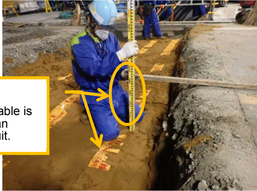
Laying a buried cable marker sheet above an underground electric line (Fukushima Daiichi NPS)
