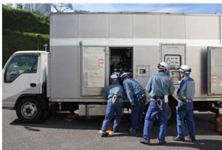
Pre-use inspection of power supply truck
