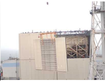
Lowering a wall panel
