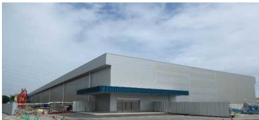
New office building (for contractors)
