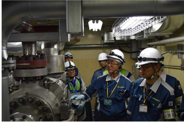
Nuclear Regulation Authority conducting field verification (Confirming installation of alternate high-pressure cooling water injection system pump)
