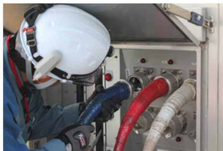
Connecting cables to a power supply truck
