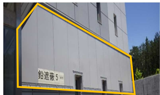
Lead panel shielding material installed on outer wall of main anti-earthquake building
