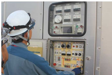
Adjusting voltage and frequency after starting up a power supply truck
