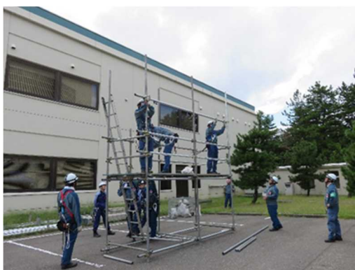
Training in assembling and disassembling scaffolding
