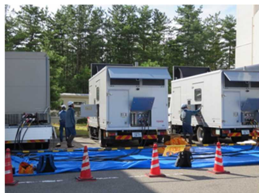
Dummy load for training in the use of power supply cars to supply electricity
