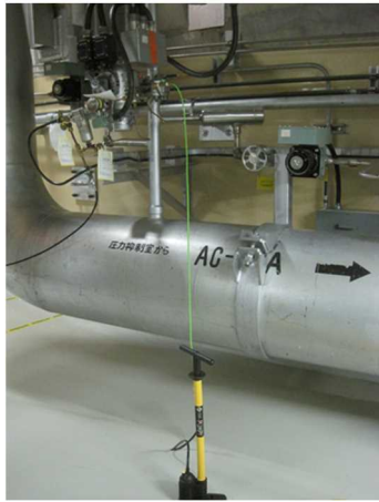
Injecting control air into an air-operated valve (left: air injection system; right: connecting operation) (Fukushima Daini NPS)
