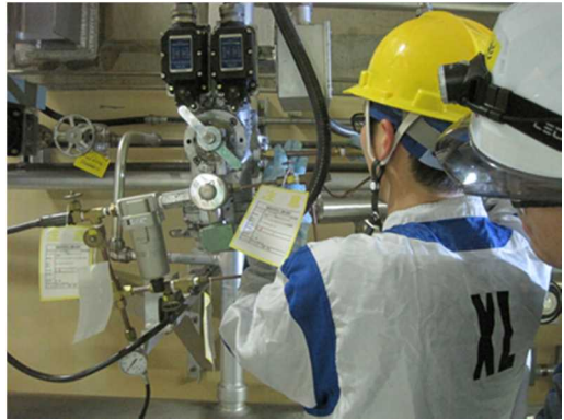
Injecting control air into an air-operated valve (left: air injection system; right: connecting operation) (Fukushima Daini NPS)
