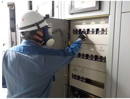
Operational training based on load reduction procedures to extend the duration of DC power sources (Kashiwazaki-Kariwa NPS)
