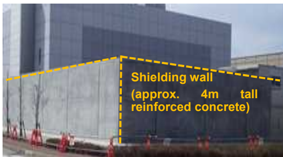
Shielding wall around main anti-earthquake building
