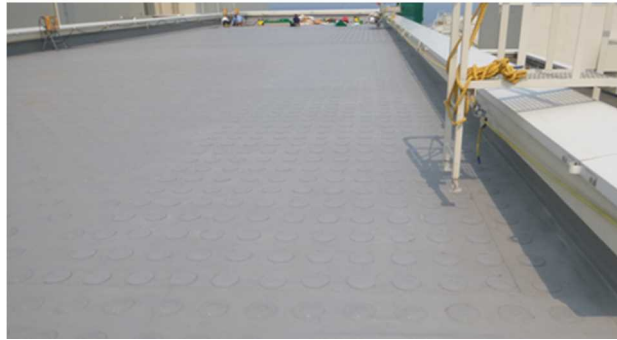
Waterproof lining applied to a building roof
