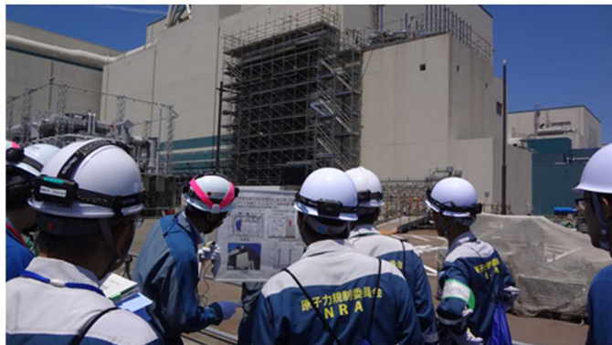
Nuclear Regulation Authority conducting field verification of filtered vent installation
