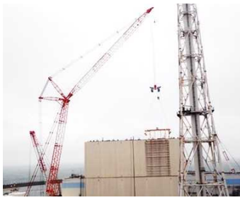
Wall panel about to be hoisted
