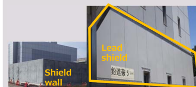
Shielding material installed on the outside walls of the main anti-earthquake building in order to prevent excessive exposure to emergency response personnel
