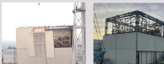
Lowering wall panels
