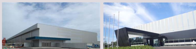
New office wing (to be used by contractors)
