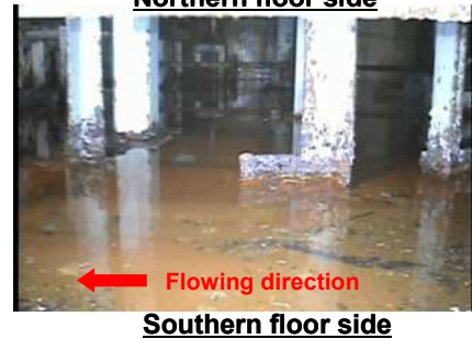
Figure 4-3 Water leaks from main steam line D in MSIV room
