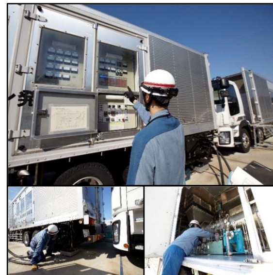
Drill to start turbine generators
