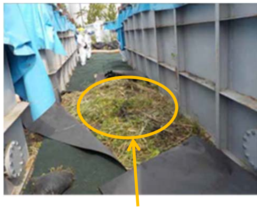
Location where piercing occurred
