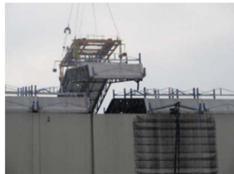
Unit 1: Dismantling roof of building cover
