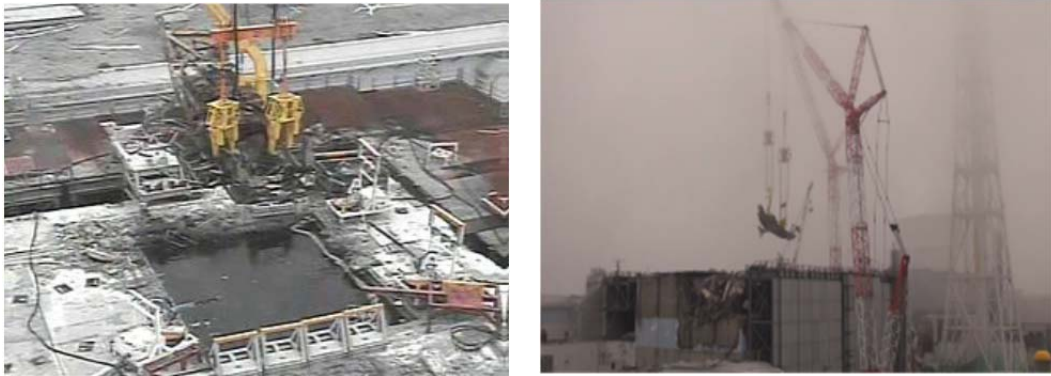
Hoisting the fuel handling machine at Unit 3
