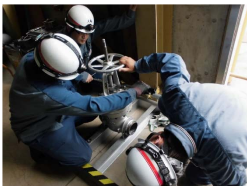
Directly managing disassembly and inspection of a valve
