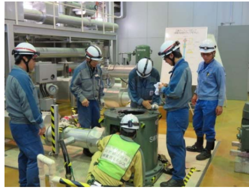
Directly managing the work to replace an electric motor on a vertical pump
