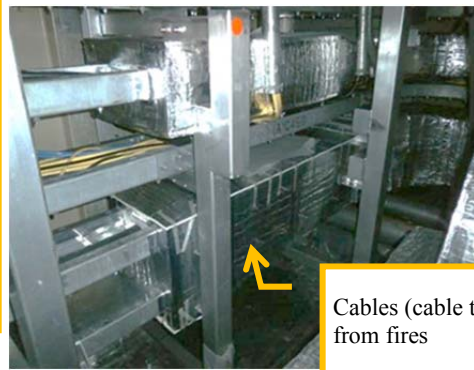
Cables wrapped for protection
