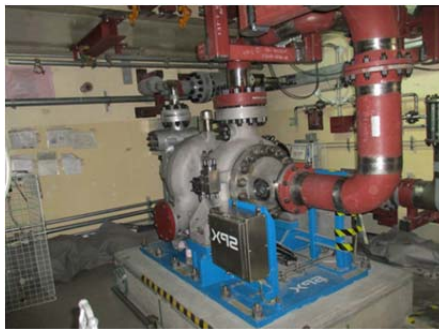
Installation of alternate high-pressure coolant injection system pump
