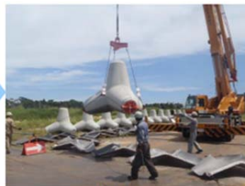
Removing block from mold
