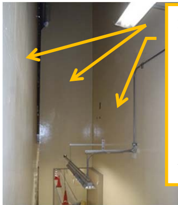
Firewalls installed (fireproof paint applied)
