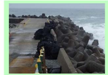
Damaged seawall at Fukushima Daiichi NPS
