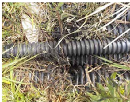
Damaged eflex pipe
