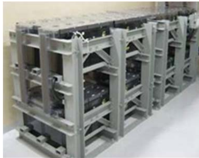
Additionally installed 125V DC storage batteries on the 4 th floor of the reactor building (encased in a seismic-resistant frame)
