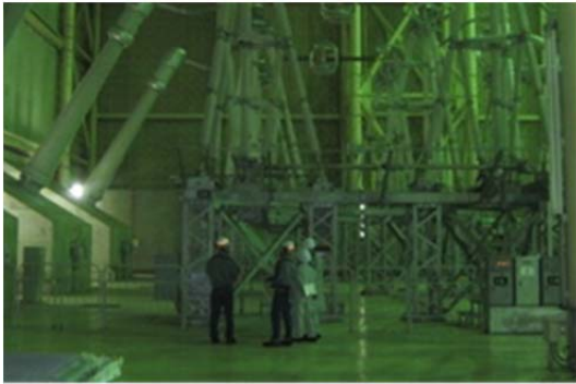
Checking switching station equipment
