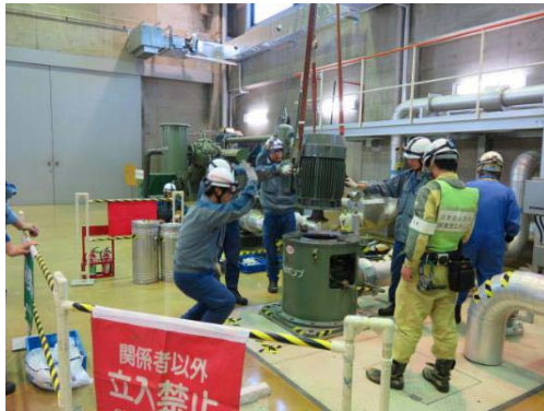
Directly managing the work to replace an electric motor on a vertical pump
