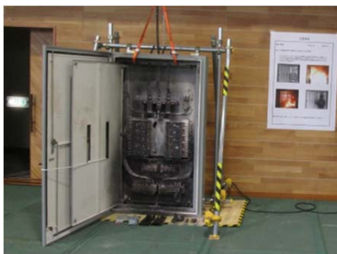
Actual switchboard displayed which caught fire and spread due to a short circuit that developed while work was being performed (presented as an example of hazards to help personnel learn about low-voltage electrical short circuits)
