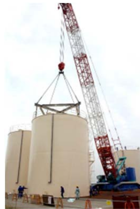
Hoisting tanks onto the shallow draft quay
