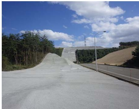
Firebreak set up within power station premises
