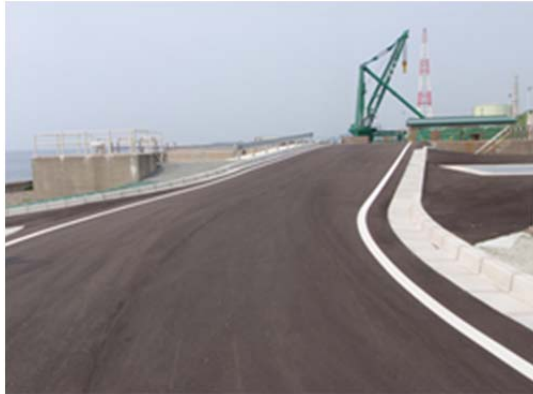
View of new access route added for travelling from Units 1-4 to Units 5-7
