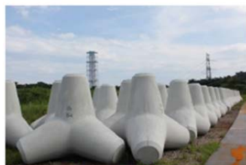
Fabricated wave-damping blocks
