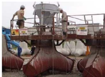
Pouring concrete into a mold
