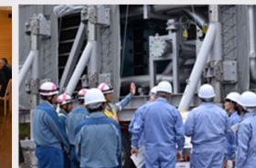
Checking safety measures facilities (Alternate heat exchanger car)
