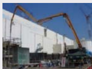
Filling Shaft at Unit 2 Seawater piping trench
