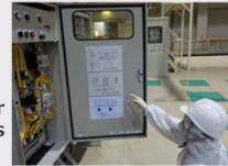
Deploying wiring diagram of seawater electric machinery for emergency responses (Fukushima Daiichi)
