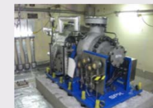
High-Pressure Alternative Cooling System (upgraded water injection function) installation
