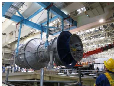
Lifting new gas turbine
