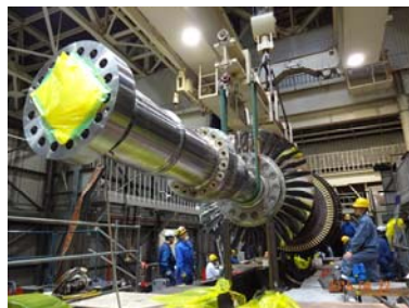
Lifting rotor of new gas turbine
