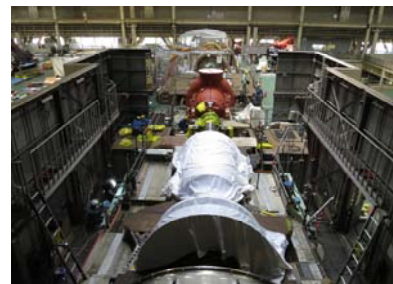
Gas turbine disassembly work
