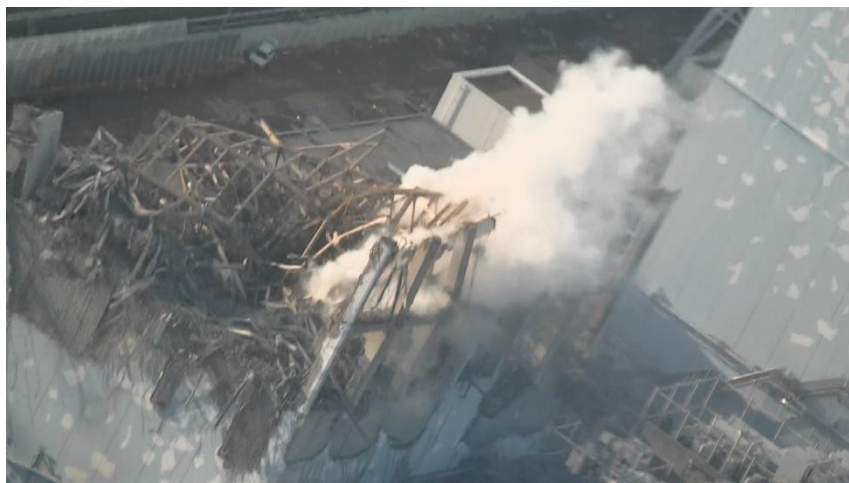
Figure 12 Aerial photo of Unit-3 (March 16 th , 2011)
