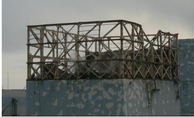
Figure Unit-1 reactor building after the hydrogen explosion
