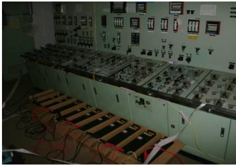
Connecting employees' private car batteries to power necessary instrumentations
