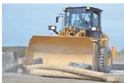
✓ Debris removal trainings
