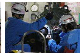
✓ Trainings to restore cooling water pumps
