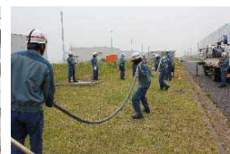
✓ Trainings to connect temporary cables
