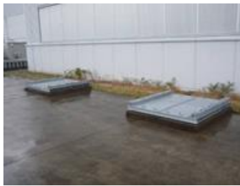
Improving water tightness of the intake channel hatches (Unit 2)
