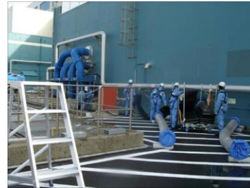
Training of connecting the alternative heat exchanger vehicle
