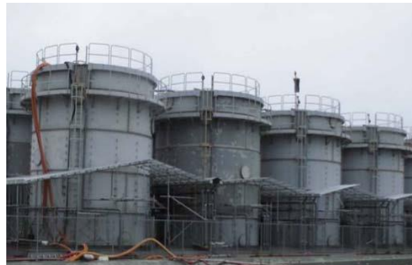
Improvement status [2]: Flange type tanks after the weir covers were installed
