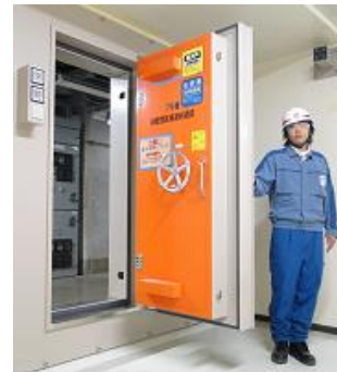
Water-tight door inside a building (Unit 7)
