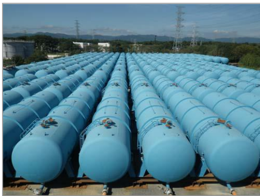
Improvement status [1]: The way tanks were installed before the improvement of H1 area
