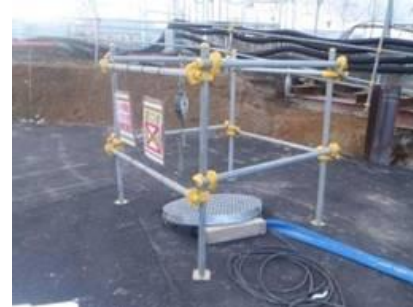
After corrective actions (Installed a barricade over the aperture)
