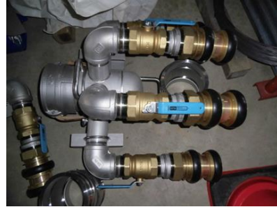
Fire hose to supply water to nuclear reactors (Kashiwazaki Kariwa)
