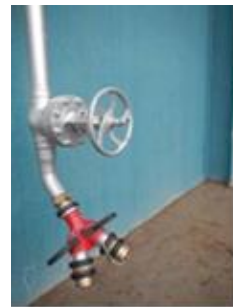
Connections to the SFP spray lines
