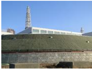
Flooding embankment (15 m high) (Oominato side)
