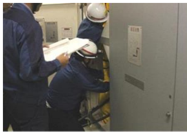
Connecting cables to the power panel
