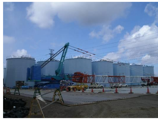
Improvement status [1]: Welded tanks installed in the H1 area
