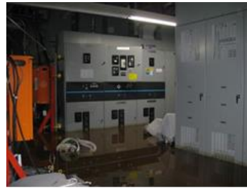
Flooding inside the building (Power room in Unit 6)
