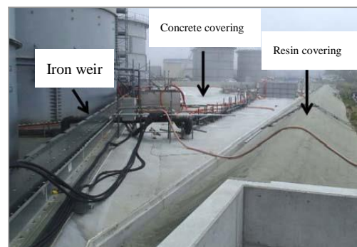
Improvement status [3]: Doubling the weir of flange type tanks and applying coating in the weir.
