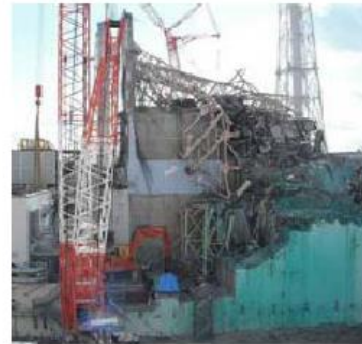
Reactor building before major debris was removed
