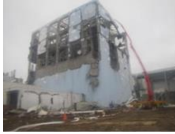
Injecting cooling water by a concrete pumping truck prepared after the accident (Unit 4)
