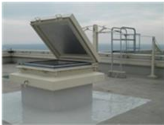
Top vent for pumping hydrogen from the reactor building (Unit 6)
