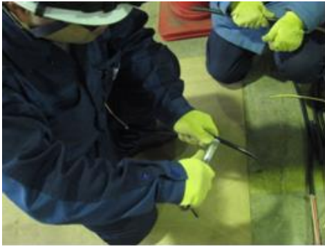
Training for handling low-tension and high-tension cable terminals at Kashiwazaki Kariwa. (Left: Sheath removal from low-tension cable. Right: Sheath removal from high-tension cable.)
