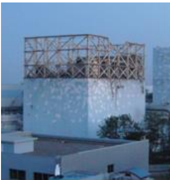
Reactor building immediately after the explosion
