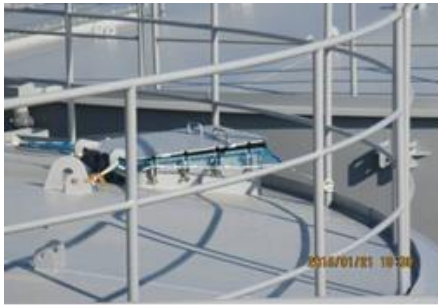
Lid of the tank with the anti-drop structure (Fukushima Daiichi NPS)
