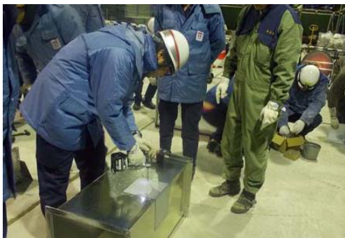
Training of air-conditioner duct emergency repair at Kashiwazaki Kariwa. (Left: Attaching reinforcing plate to cracked portion. Right: Making periphery of the reinforcing plate airtight with repair tape.)
