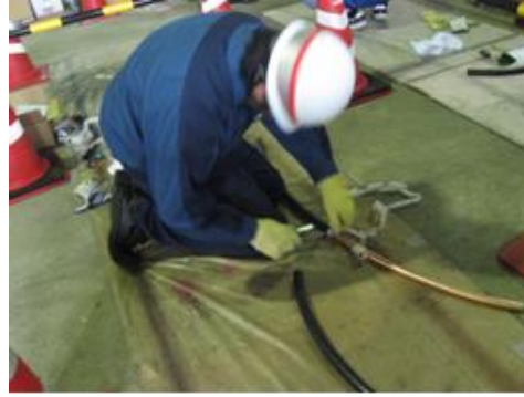
Training for handling low-tension and high-tension cable terminals at Kashiwazaki Kariwa. (Left: Sheath removal from low-tension cable. Right: Sheath removal from high-tension cable.)
