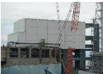
Reactor building after installing the fuel removal cover
