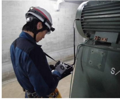
Data collection by direct management of operator (Diagnosis of motor vibration)
