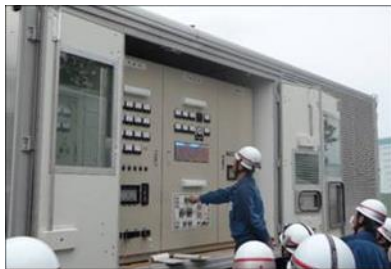
Conducting a startup test on a gas turbine generator
