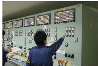
Conducting training in the main control room
