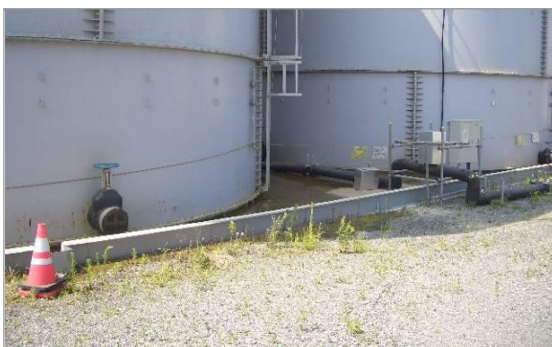
Improvement status [3]: Circumference of weir of flange type tanks before the improvement
