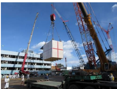
Installing the measuring equipment
