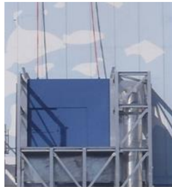
Aperture of the closed blow out panel
