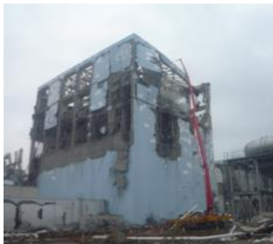
A concrete pumping truck injecting cooling water into the fuel pool immediately after the accident
