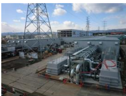
Freezer plant building where freezers are installed
