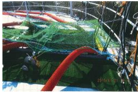
Anti-drop measure against the aperture of the hatch (Fukushima Daiichi NPS)
