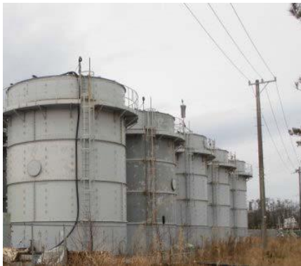
Improvement status [2]: Flange type tanks before the improvement
