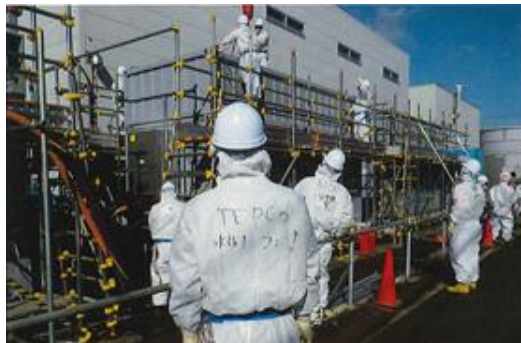
Installing mobile-type strontium removal equipment (At Fukushima Daiichi NPS)
