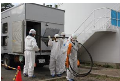
Pulling out cables from the power supply car
