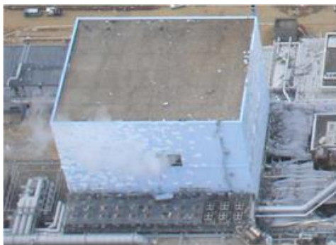
Reactor building with the blow out panel opened immediately after the accident
