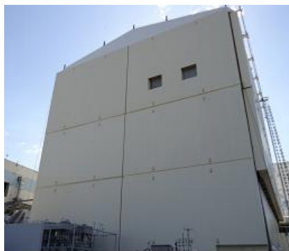
Covered reactor building
