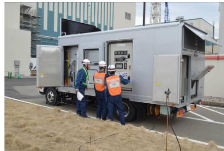
Power supply sharing drill by a power supply car
