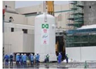
Filtered vent equipment (Unit 6)
