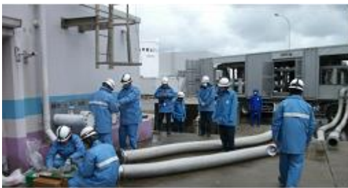
Training of connecting the alternative heat exchanger vehicle
