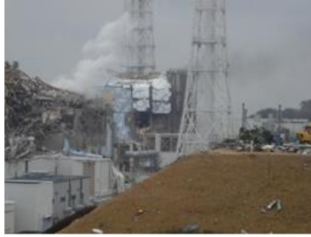
Reactor buildings of Units 3 and 4 after the hydrogen explosions
