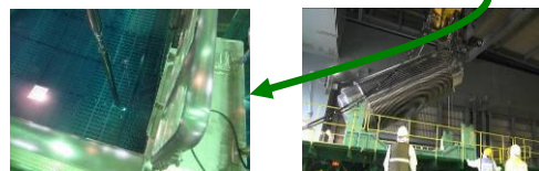
Preparations to remove fuel from the spent fuel pool
