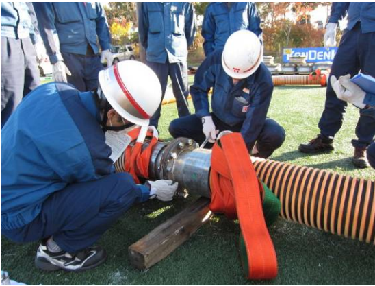
Temporary hose (Kanaflex) connection drill at Fukushima Daiichi (Left: Hose to hose connection, Right: Connection to different diameter flange)
