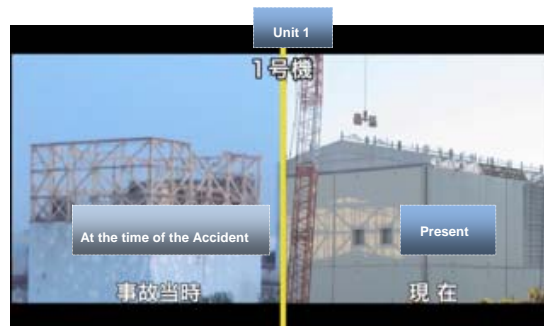
A scene of the video “Current Fukushima Daiichi Nuclear Power Plant”
