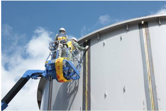
Welded part inspection
