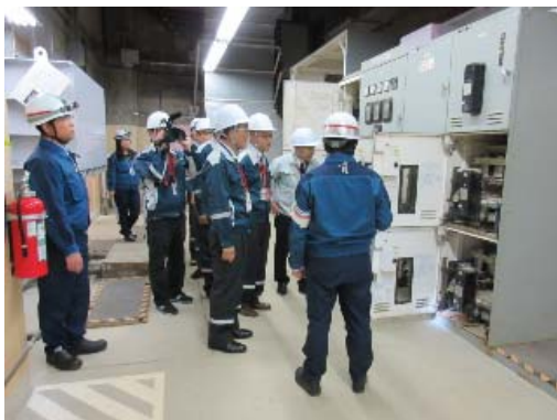
Power distribution panel submerged by tsunami (Unit 1)
