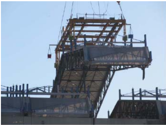
Removal of roof covers/panels from Unit 1 reactor building
