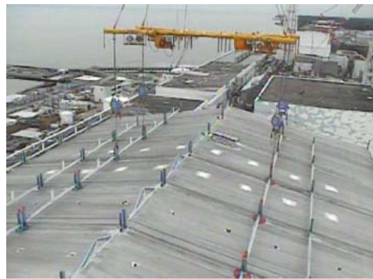
Reinstallation of roof panels after investigation
