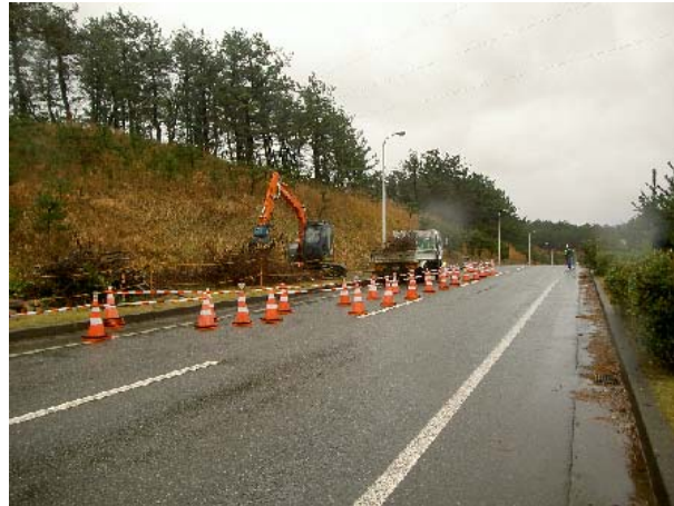
Installation of a firebreak
