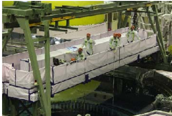
Inspection of the structural substances in the reactor (Lowering an underwater camera into the reactor)
