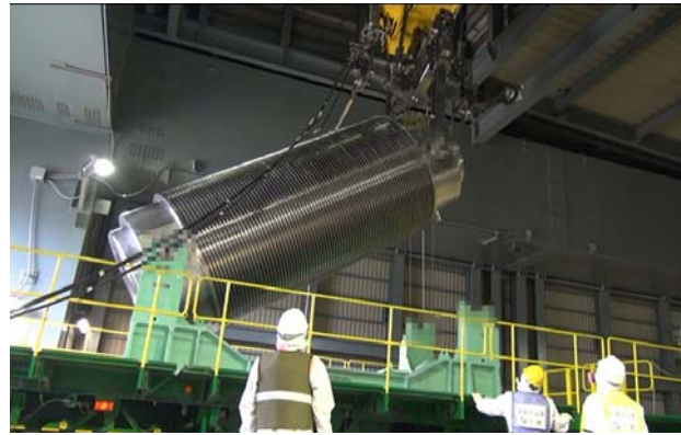
Loading of transportation container from on-site to trailer
