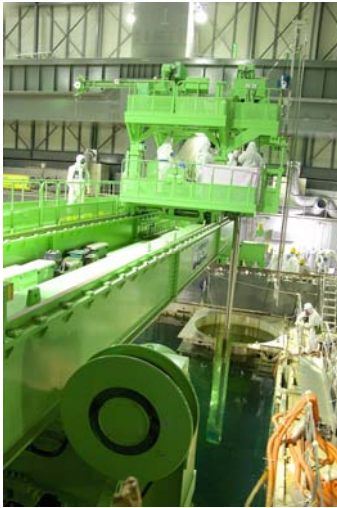
Status of fuel removal
