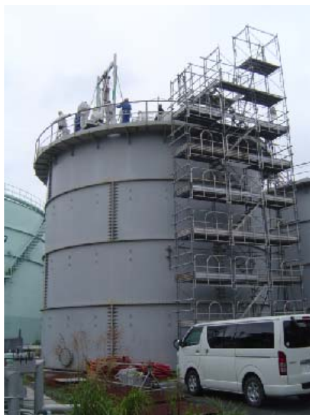
Flange type tank where the demonstration test is performed
