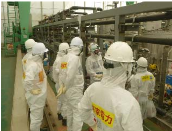
Advising and instructing on-site workers regarding installation of high-performance multi-nuclide removal equipment
