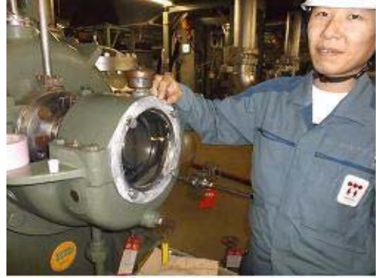
Establishment of restoration procedure for the pump penetrated by seawater (Fukushima Daini) (Cover (clear) temporarily placed for simulation of submersion)
