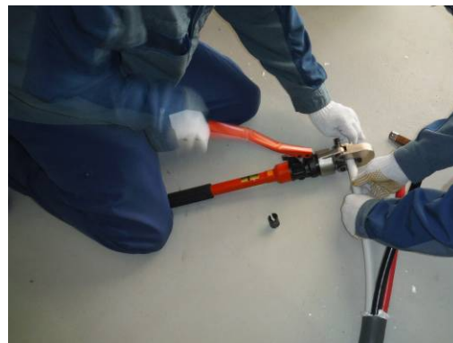
Training for handling low-tension cable terminals
