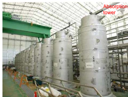
Installation of high-performance multi-nuclide removal equipment
