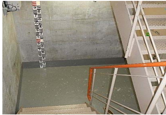
Installation of a simple measure for understanding the level of submersion (Kashiwazaki Kariwa)
