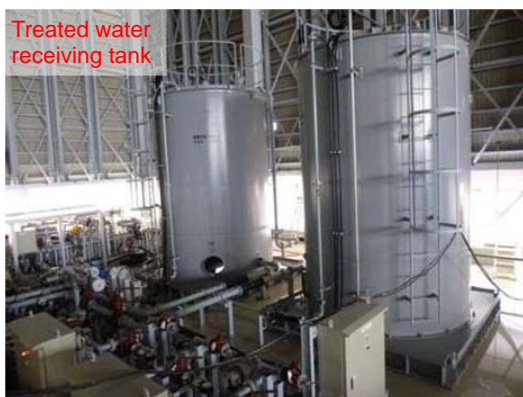
Installation of extended multi-nuclide removal equipment
