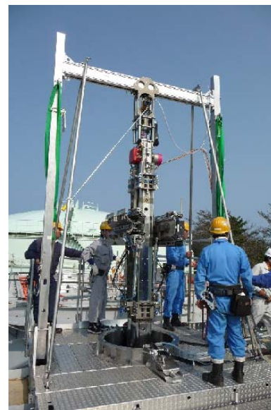
Training for repairing the flange on the bottom of the tank
