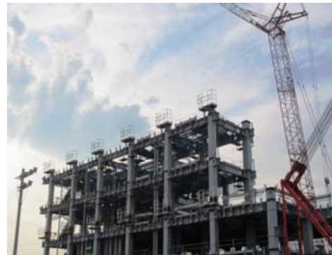
On-site large-scale rest facility that is under construction
