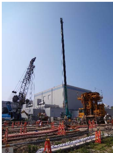
Operation of examining the shaft in the side of Units 1 to 4
