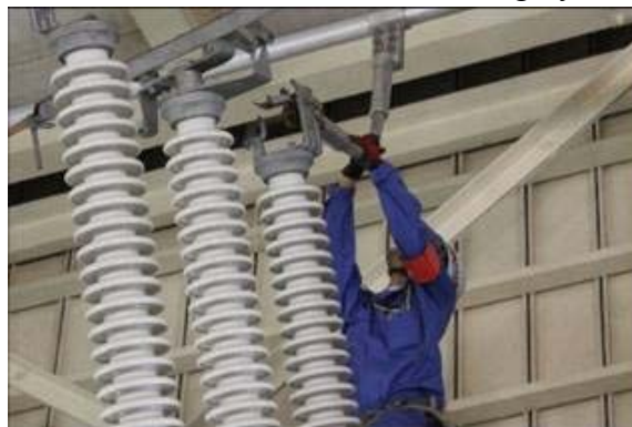
Inspection of the power supply line of 66,000 volts
