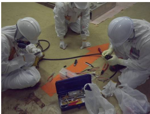
Training for handling low-tension cable terminals
