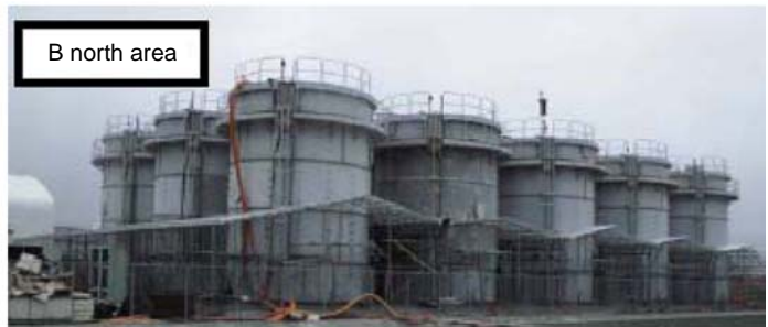
Installation of weir covers (ceiling material)
