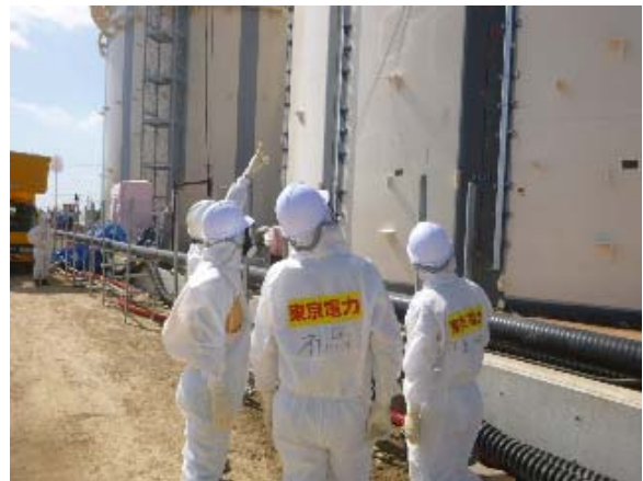
Checking operation status of tank installation in J4 area
