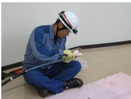
Training for handling high-tension cable terminals
