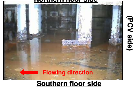
Figure 4-3 Water leaks from main steam line D in MSIV room
