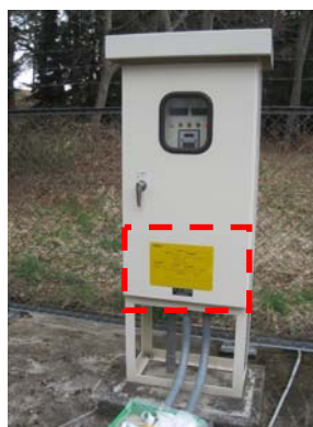
Pasting the system outline diagram on the deep well No.1 pump control panel
