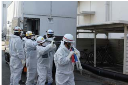
Pulling out cable from power source vehicle
