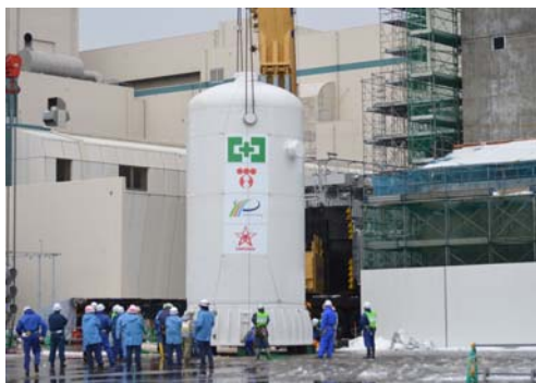
Unit 6 Installation of filter vent unit
