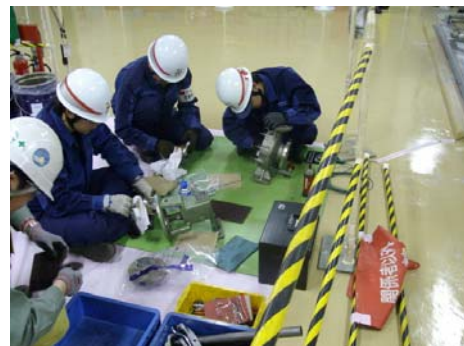
Disassembly of pumps and parts maintenance
