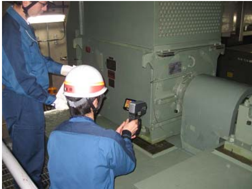
Equipment diagnosis by operators (Example: Infrared thermography diagnosis)
