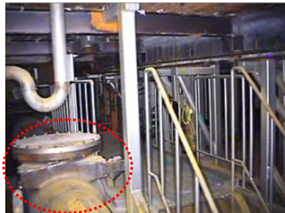
Figure 2-3 Camera photo of an S/C vacuum breaker in the torus room of Unit-1
