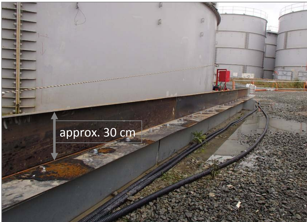
Dikes with steel plating installed (H4 north)
