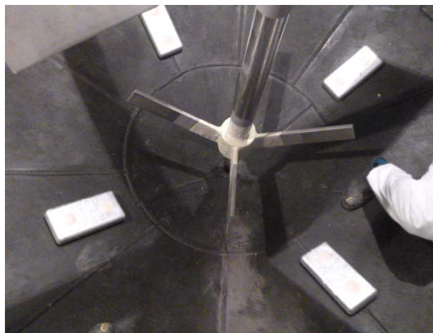
Batch treatment tank 1C (after rubber lining attached)
