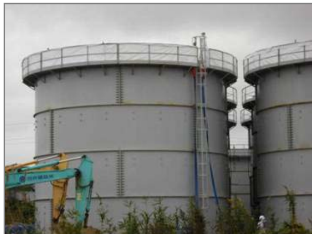
Full view of tank
