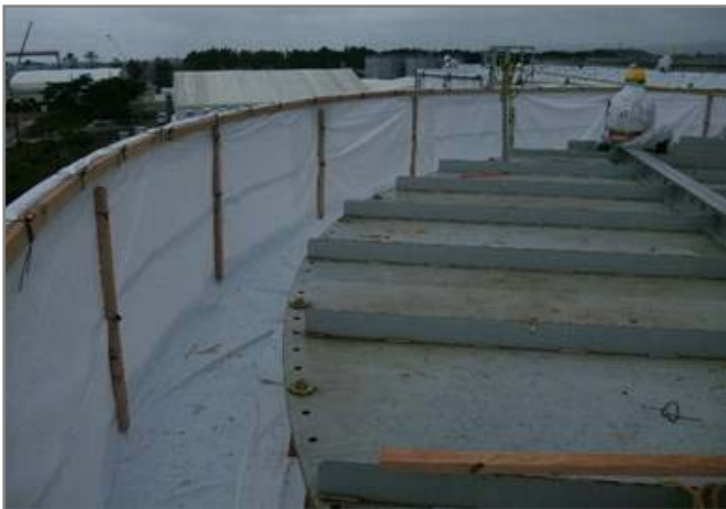
Tank inspection platform
