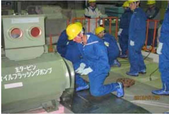
Work for replacing an electric motor
