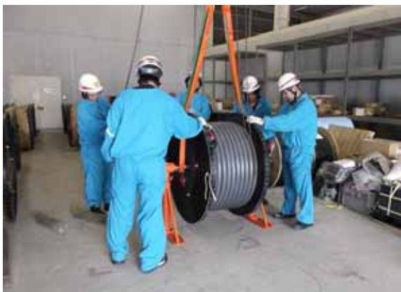
Work laying temporary cable
