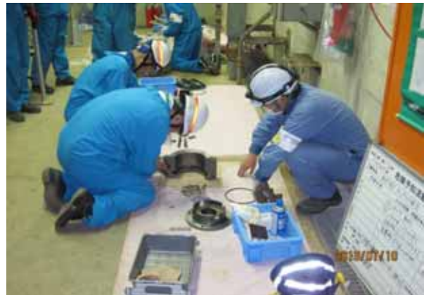
Work restoring a cooling pump
