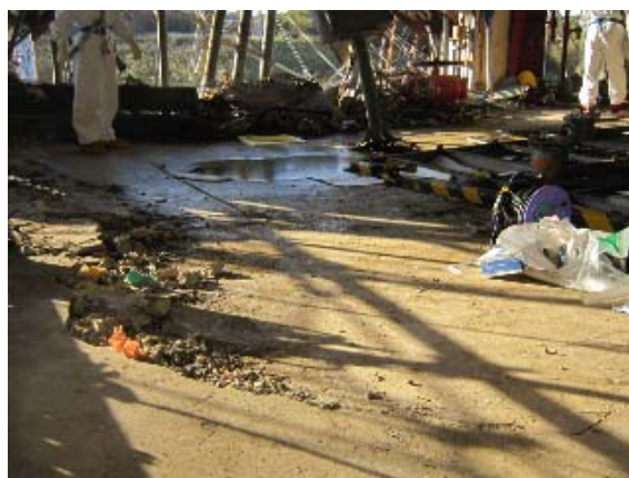
Investigation of condition of 4 th floor of Unit 4 R/B Floor surface has caved in, and it is estimated that the explosion occurred on the 4 th floor. (November 10, 2011)
