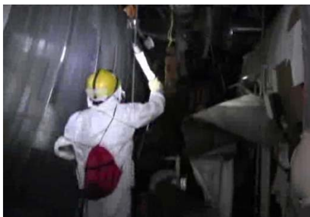
Investigating the side of isolation condenser unit at Unit 1 (October 18, 2011)
