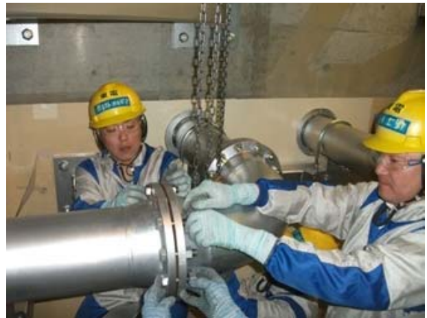
Work to connect a replacement heat exchanger
