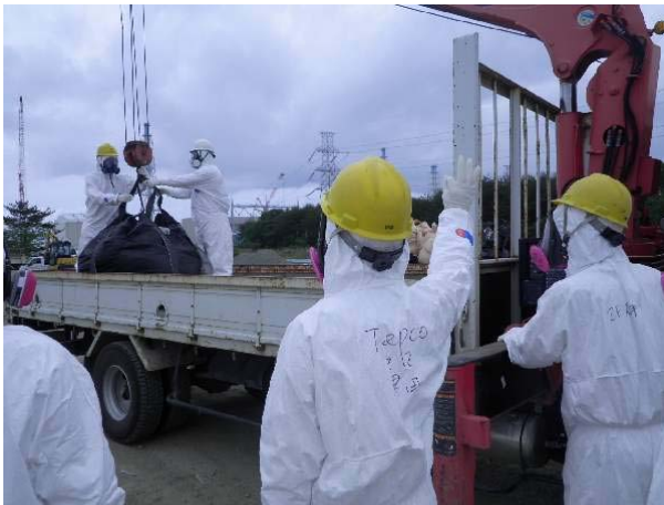
Unloading work performed using vehicle equipped with a crane
