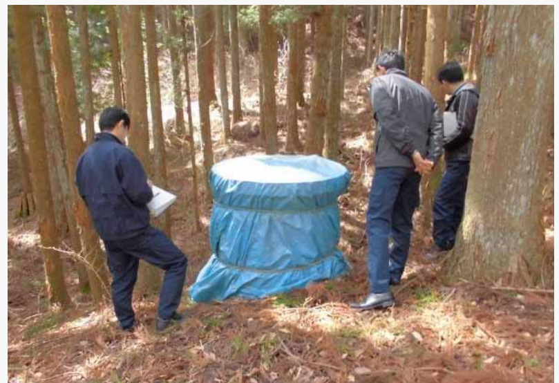
<Photo> Site survey of existing well in Katsurao Village
