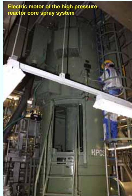
Trial operation [Permanent installation completed on March 25, 2013] (Photo taken on March 25, 2013)
