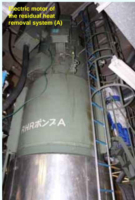
Trial operation [Permanent installation completed on March 15, 2013] (Photo taken on March 15, 2013)
