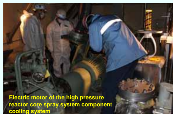
Trial operation [Permanent installation completed on March 14, 2013] (Photo taken on March 14, 2013)
