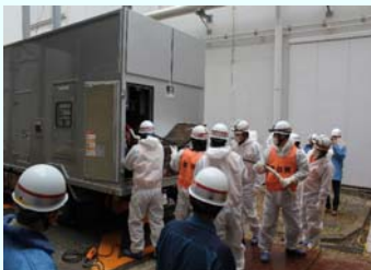
Pulling out cable from a power supply car (Unit 2)
