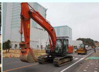
Checking the access route at the site (around the Reactor Building)
