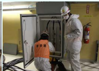
Making connection with the cable connection box (Unit 2)
