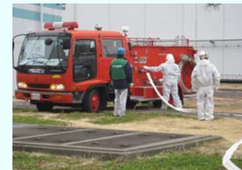
Preparing to transfer water to the Reactor Building (Unit 2)
