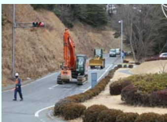
Heavy machinery heading to the site
