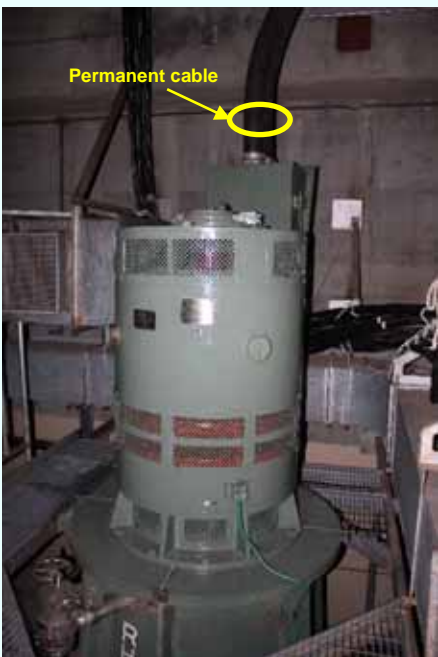
Switching to the permanent cable completed (Photo taken on February 8, 2013)
