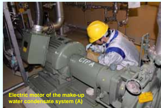
Trial operation [Permanent installation completed on February 7, 2013] (Photo taken on February 7, 2013)
