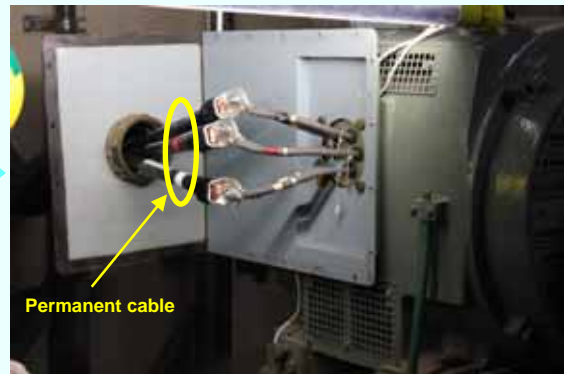
Switching to the permanent cable completed (Photo taken on February 7, 2013)
