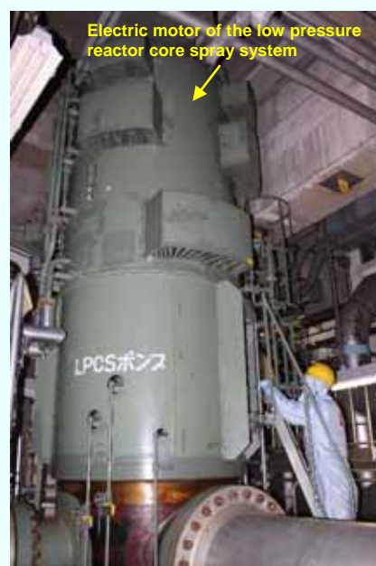
Trial operation [Permanent installation completed on February 23, 2013] (Photo taken on February 23, 2013)
