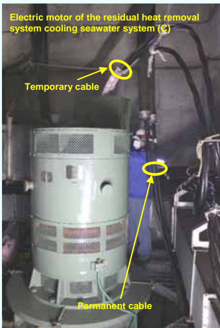
Before switching to the permanent cable (Photo taken on February 8, 2013)
