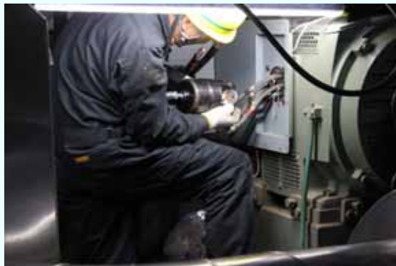
Installation of the permanent cable terminals (Photo taken on February 7, 2013)
