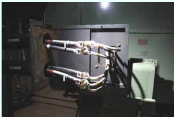
After permanent cable installation (Photo taken on January 25, 2013)
