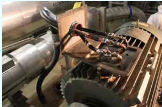
After permanent cable installation (Photo taken on January 21, 2013)
