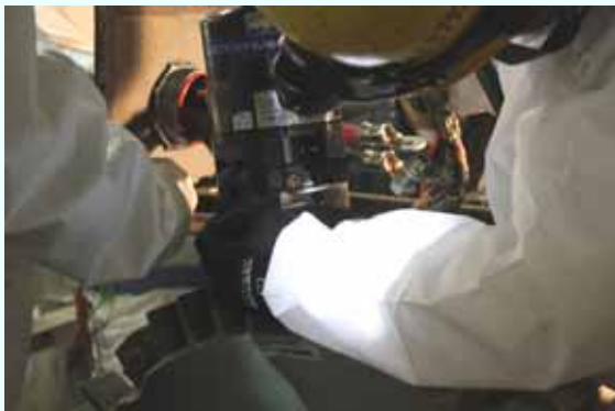
Terminal installation for the permanent cable (Photo taken on January 21, 2013)
