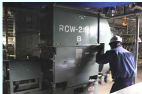
Trial operation [Permanent installation completed on January 29, 2013] (Photo taken on January 29, 2013)
