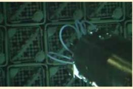
Fuel assembly being inserted into the spent fuel rack (2)
